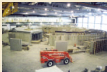
Booster Ring Structure —Under Construction
